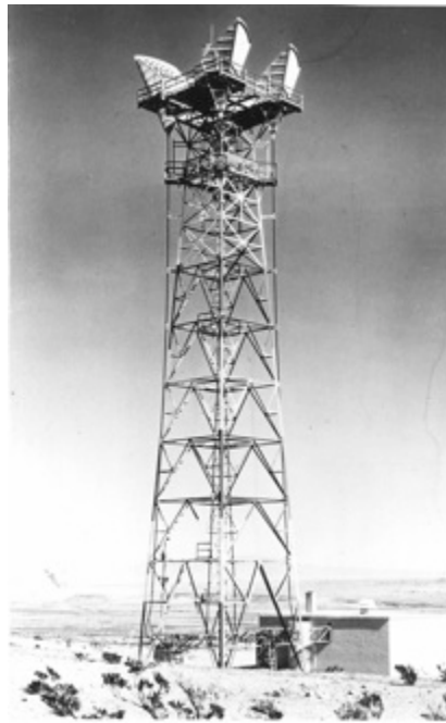
Fig. 5-12. Long-distance telephony utilized a series of microwave towers about every 26 miles to relay signals across the United States. The horn antenna, invented at Bell Labs, allowed radio waves to be polarized and doubled the capacity of earlier systems. [1962 photo courtesy of Alcatel-Lucent USA Inc. / Bell Labs.]
