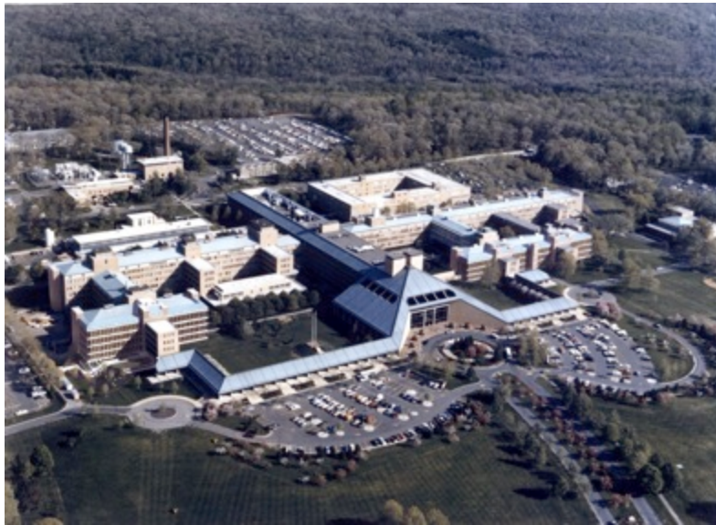
Fig. 2-5. Buildings 6 and 7 at Murray Hill were completed in 1974 and were situated between Buildings 1 and 2, replacing what used to be a Concourse. Building 7 was to the rear; Building 6 with its pyramid-like structure was to the front and became the main entrance to Bell Labs. Two covered walkways extended to the sides of the pyramid, like welcoming arms. Executive offices and the library were in the pyramid structure of Building 6. This dramatic aerial photograph is from the early 1980s. [Photo courtesy of Alcatel-Lucent USA Inc. / Bell Labs.]
