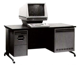
Tektronix has merged two significant graphics technologies to create a technological first. The new 4081 Interactive Graphics Terminal is a picture manipulation tool with potential for more productive man/machine interaction. Refresh tube technology provides motion; storage tube technology offers high-resolution graphics, even of complex images.
