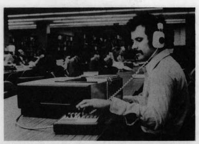
Fig. 1-5. A desktop reading machine (courtesy of Kurzweil Computer Products).
