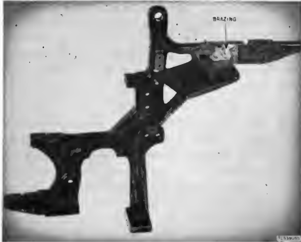
Figure 131. Repair by brazing.
