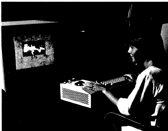
Figure 3—Interactive extraction of lakes from LANDSAT imagery achieved through utilization of the COMTAL display and associated trackball/cursor unit. (JPL Photo Lab Negative No. 324-2287Ac)
