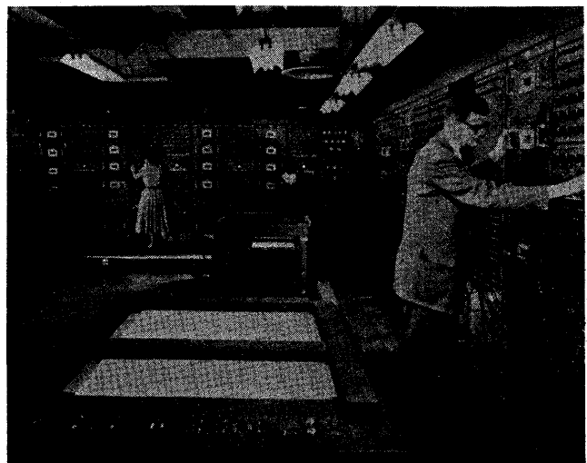
Figure 8—Reeves computer installation, courtesy Reeves Instrument Company
