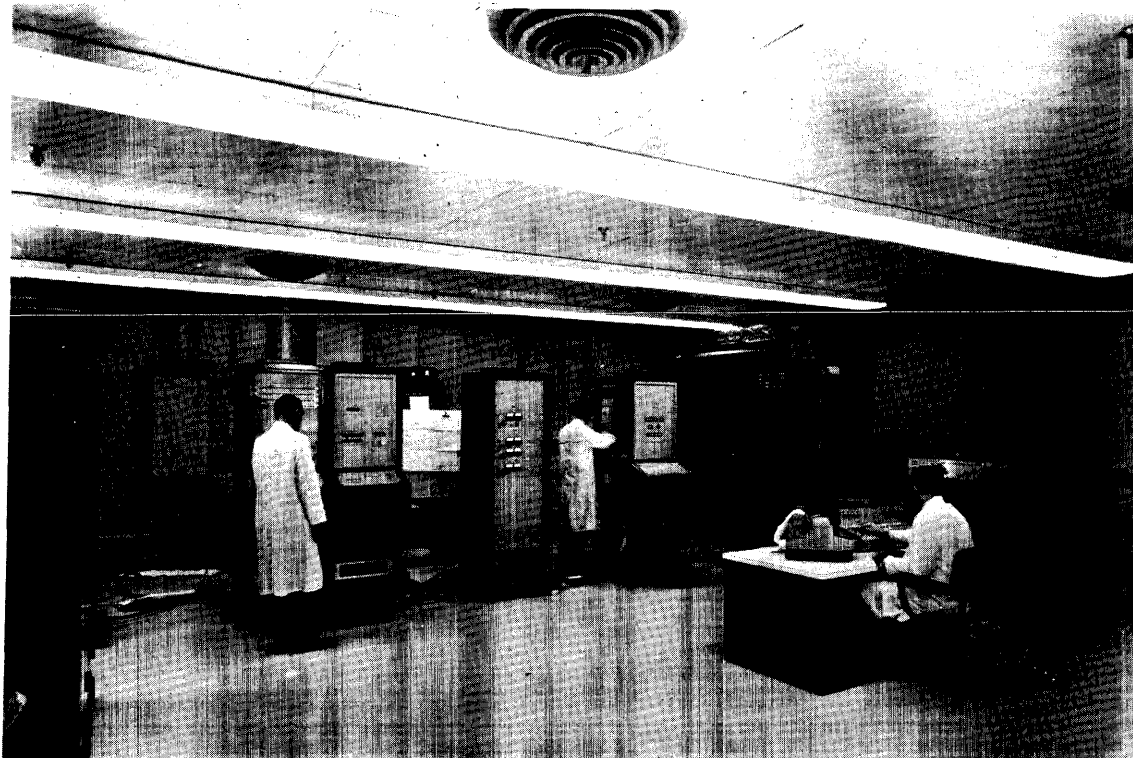
Figure 9. Ground operation equipment at a typical remote control station.
