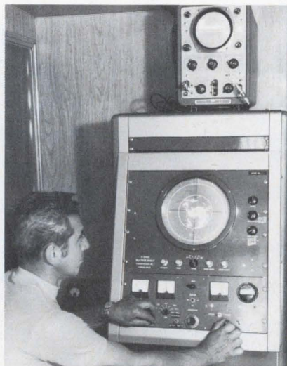
Clouds show up as shadowy images on the screen of a radar that will be used in the country's first large-scale operational water-making project, starting this winter in southern Colorado under the auspices of the Bureau of Reclamation, Boulder, Colo.
