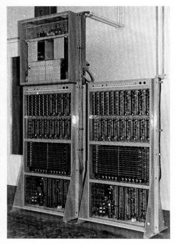
The two Pentaconta CM 12 concentrators installed in the Paris regional telephone network.
