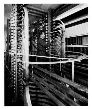
Switching facilities for pneumatic tube distributing system that handles toll tickets without carriers.
