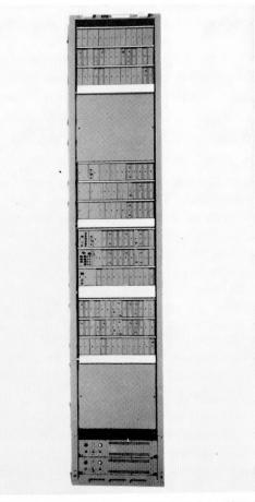
Figure 22—Master and supermaster groups for a 2700/ 1800-channel telephone system are mounted in this bay, which is 520 millimeters (21 inches) wide and 2750 millimeters (108 inches) tall. Design conforms with the standard equipment practice for ITT Europe.
