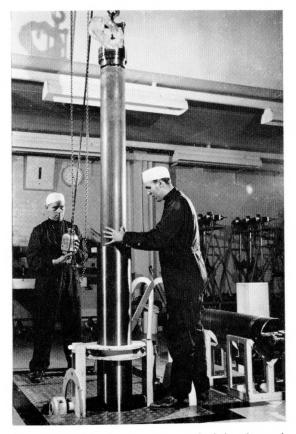
Figure 5—Telephone repeater capsule being lowered into the high-strength steel case that can withstand sea-bottom pressure preparatory to undergoing testing before being accepted for service.
