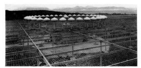
Figure 16—Circular array of 39 radiators for the Doppler very-high-frequency omnidirectional radio range near Salzburg, Austria.
