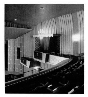
Figure 15—Column loudspeakers built into proscenium arch.
