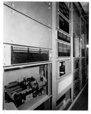
Figure 7—Madrid-Almagro toll exchange test and traffic control bays. A punched-card machine is shown at the lower left.
