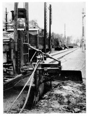
Figure 12—Plowing the cable into the ballast of the railway line.
