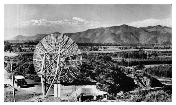
Figure 5-Receiving antenna at Naltagua Bridge site.
