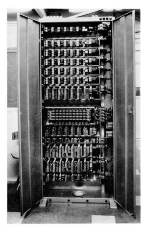
Figure 3—Small rural exchange with 32 subscriber lines connected.
