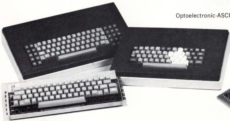
Micro Switch keyboards with 63-key ASCII MOS encoding (foreground), 78-key ASCII DTL encoding (top), and 51 key EBCDIC MOS encoding.
