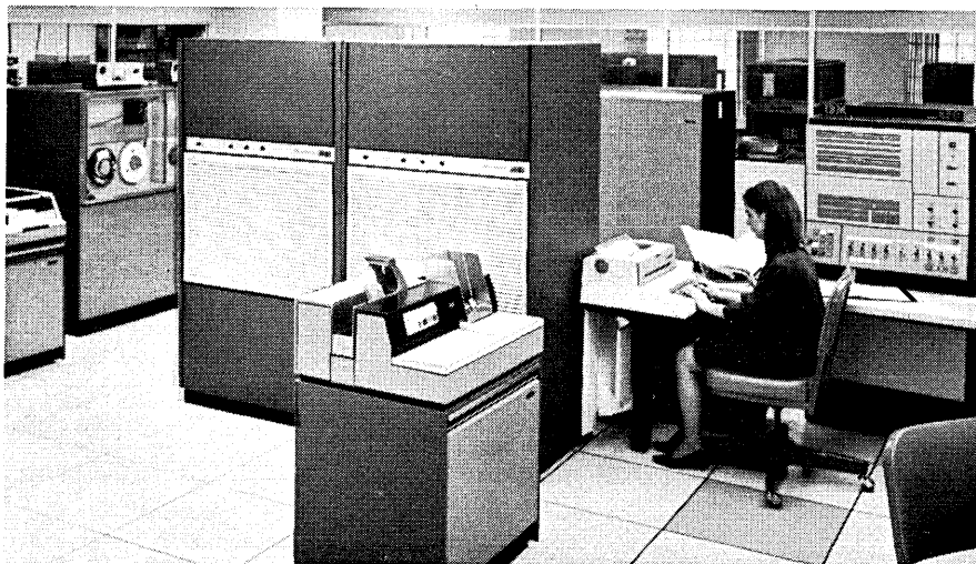
Twin 5-ton units on location
