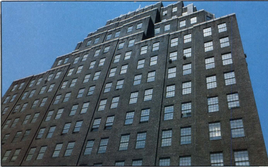
Sylvan-Lawrence, owner of the Port Authority building (above), was also the contractor that built CSC's data center. One hundred employees work in the center, 30 of which are professionals.
