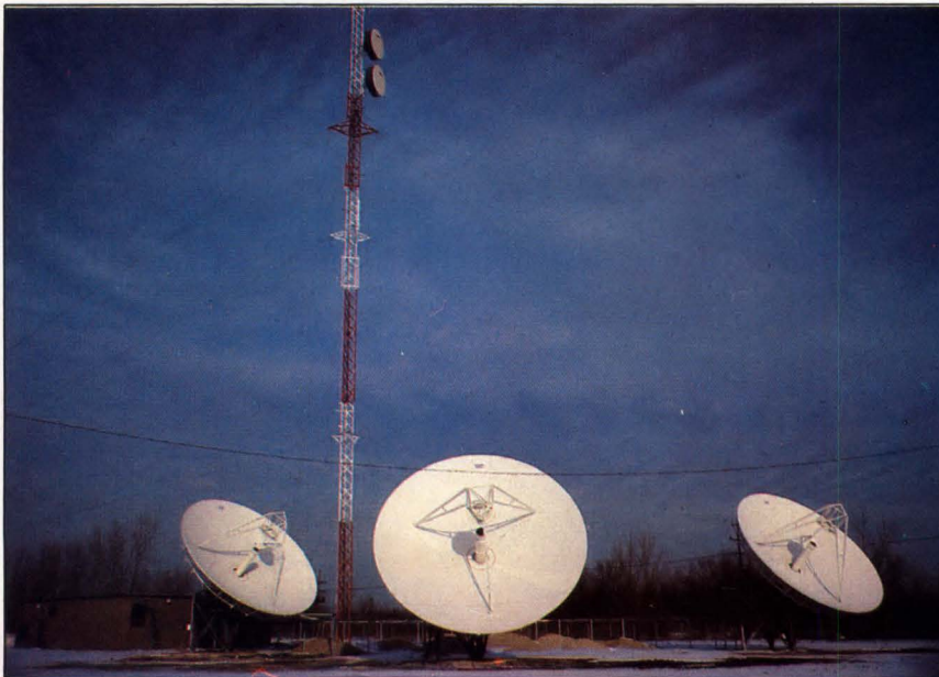
The earth station of the Chicago Teleport is located in Skokie, IL, 10 miles removed from the interference-loaded airwaves of the Windy City. Signals are transmitted to the station via repeaters.
