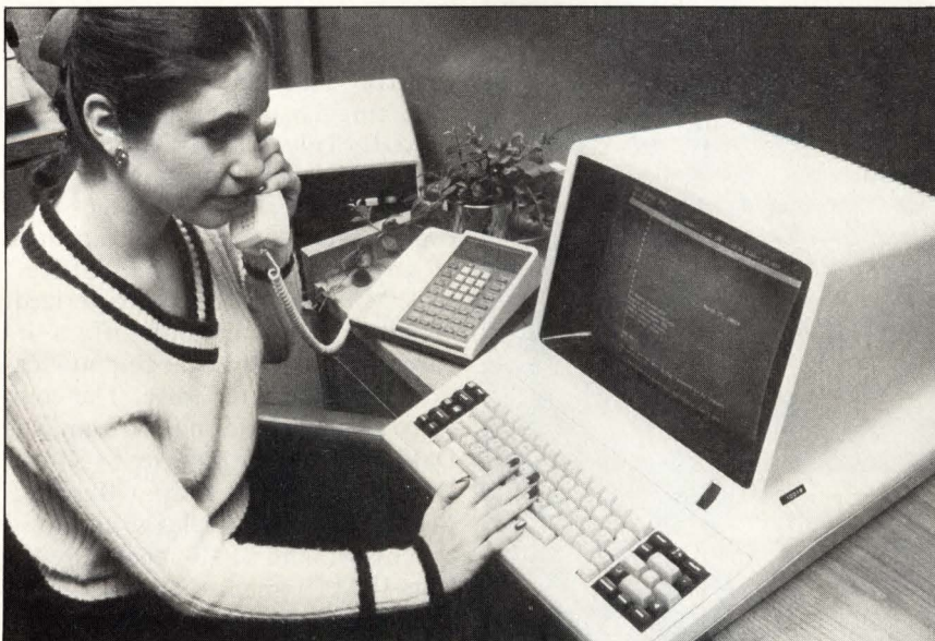
This operator is accessing a Lexar private automatic branch exchange that is part of an internal communications utility in her employer's building. The system was built by United Technologies' Building Systems Co.
