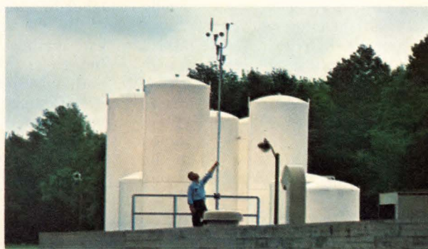
This weather station is a key part of a sensor-based heating and cooling system at IBM's East Fishkill facility.
